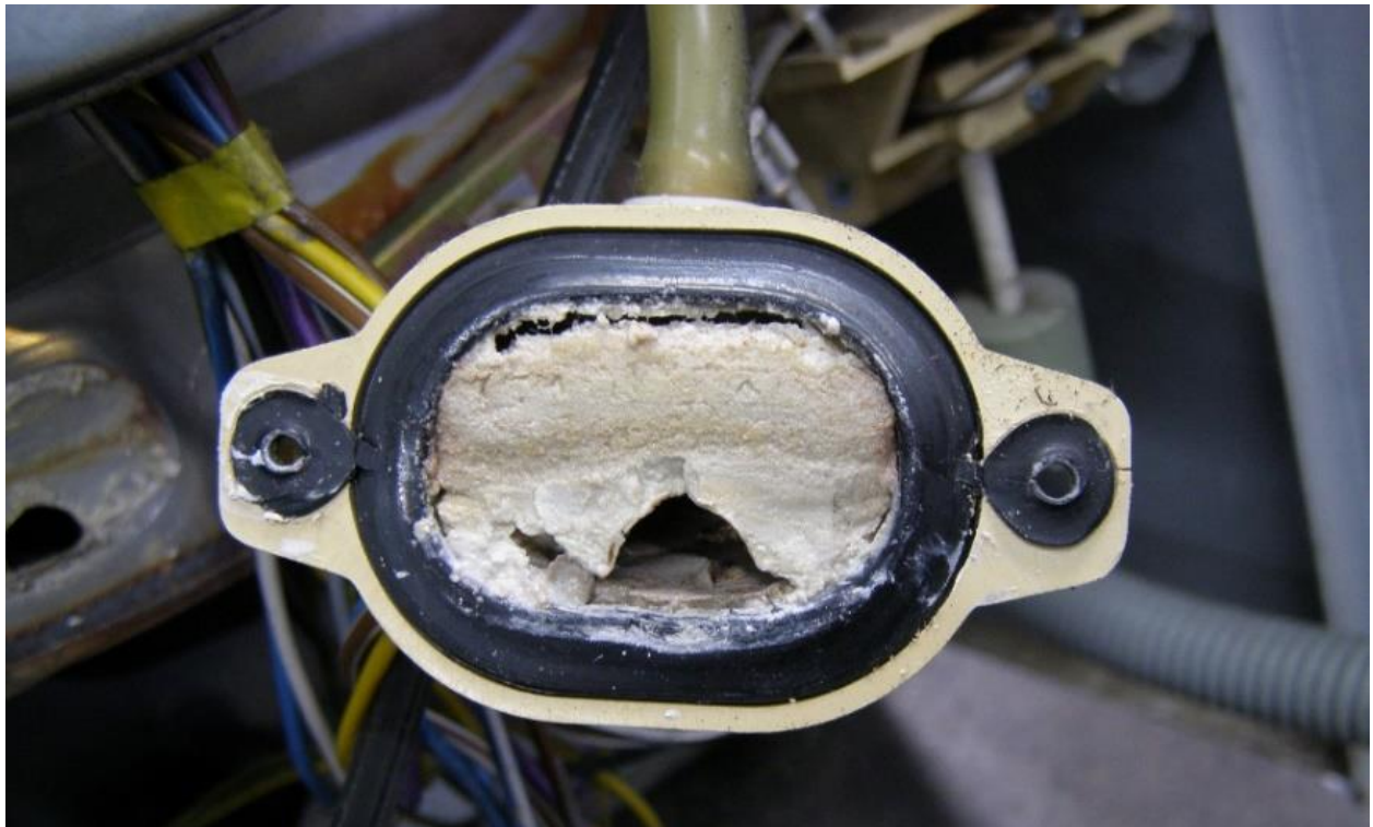
Figure 3.20. Blocked pressure chamber, possibly as a result of calcification and detergent overdose
